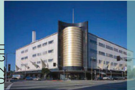
The May Company building will house a movie museum.
