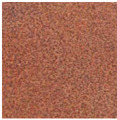
Rust Grade C
