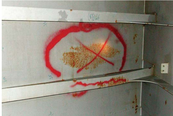
Photograph 12-22. Reverse impact from external collision.
