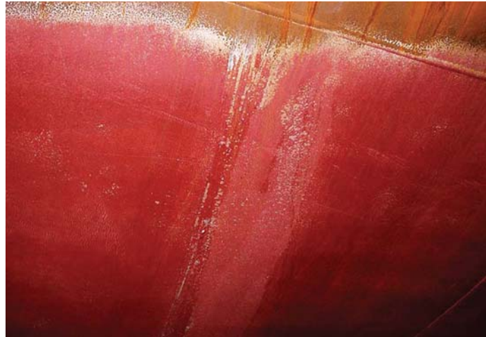
Photograph 12- 6. Washing was occurring on the area above the wet paint and the washing water caused coating removal.
