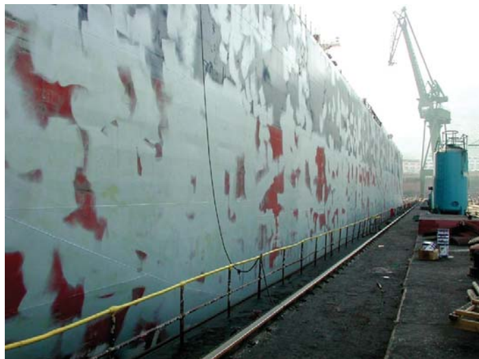
Photograph 4-1. Outer hull showing application of primer after localized spot blasting.
