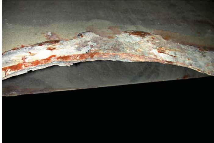
Photograph 12-18. Well performing cathodic protection system, with tight calcareous deposits.
