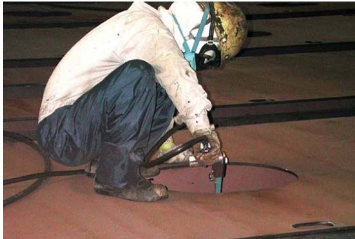
Photograph 4-6. Edge preparation using a belt grinder.
