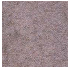
C HB 2 Rust Grade C Hydroblasted to an Sa 2 equivalent
