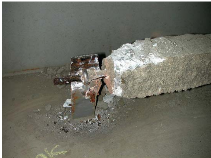
Photograph 6-1. Normally working anode.
