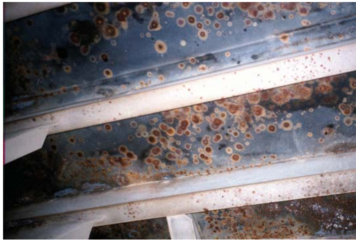
Photograph 12-9. Through film breakdown.
