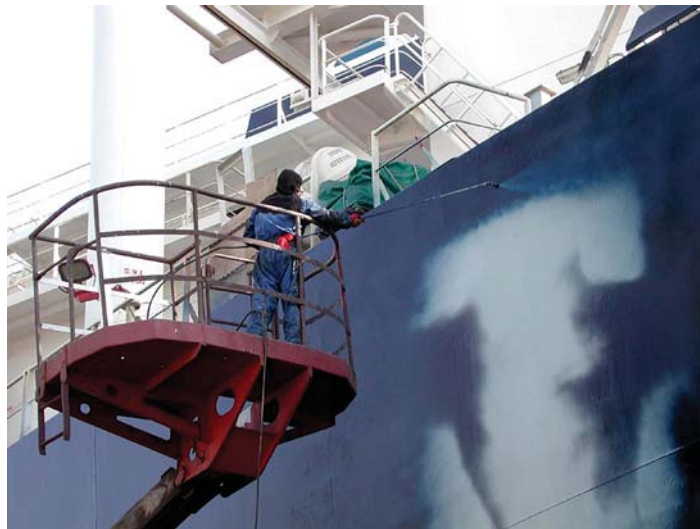
Photograph 5-3. Airless spray application of paint onto the vessel's topsides.
