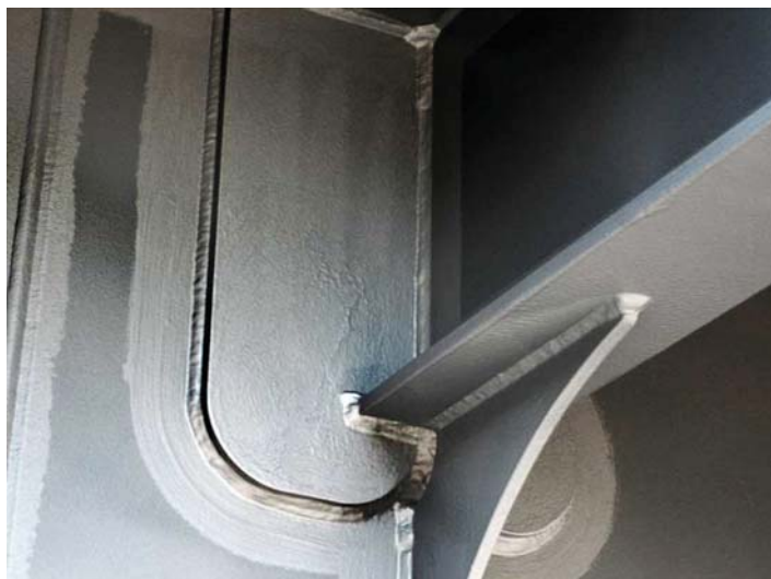
Photograph 5-2. Stripe coating on welded details.
