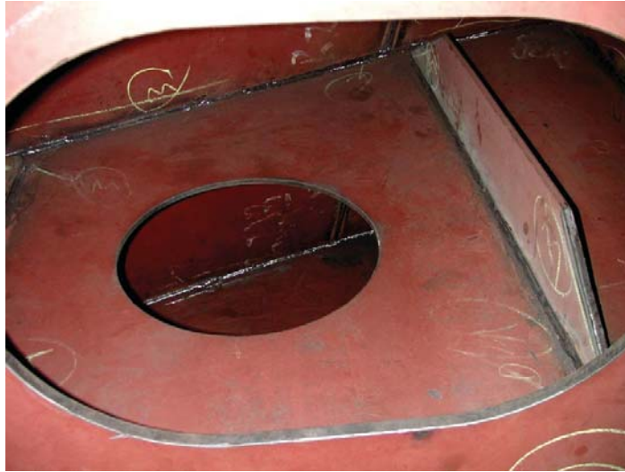
Photograph 4-11. Complex structure, with lower welds only accessible through the hole.
