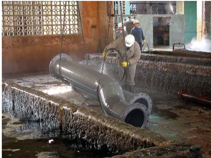
Photograph 4-8. Pipes undergoing pickling.
