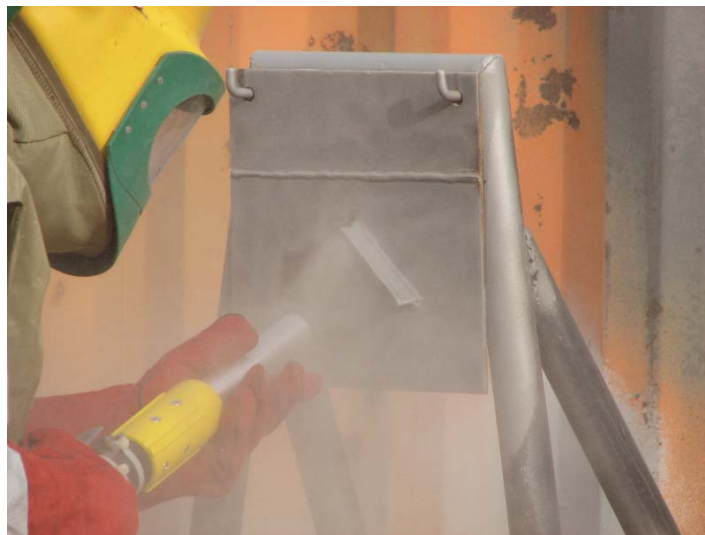
Photograph 4-4. Abrasive blasting.
