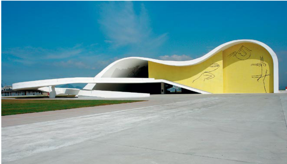
Vista exterior fachada principal
