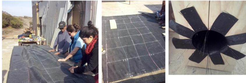
Drawing and fixing the geotextile to the rigid matrix of the formwork with glue and staples.
