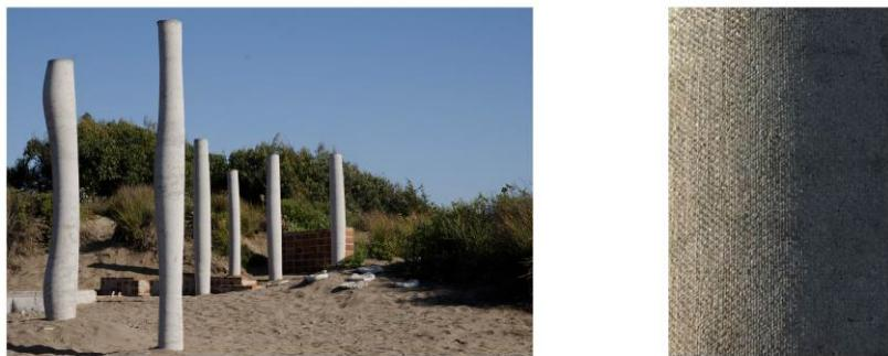
Columns are a basic architectural element: with flexible formwork it is possible to achieve new forms for them.
