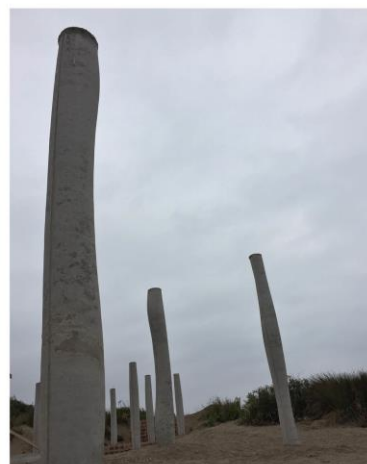
The seventeen built columns in situ.
