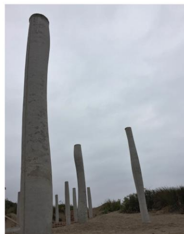
The seventeen built columns in situ.
